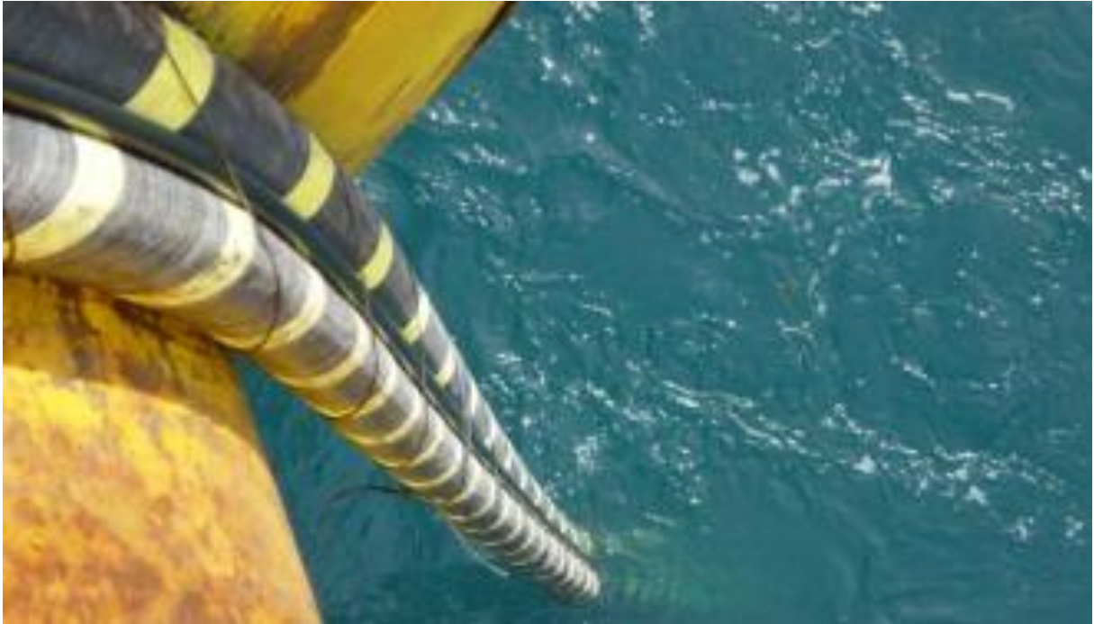
Figure 2. Typical bundled HVDC cable cores and a smaller fibre optic cable during installation.
