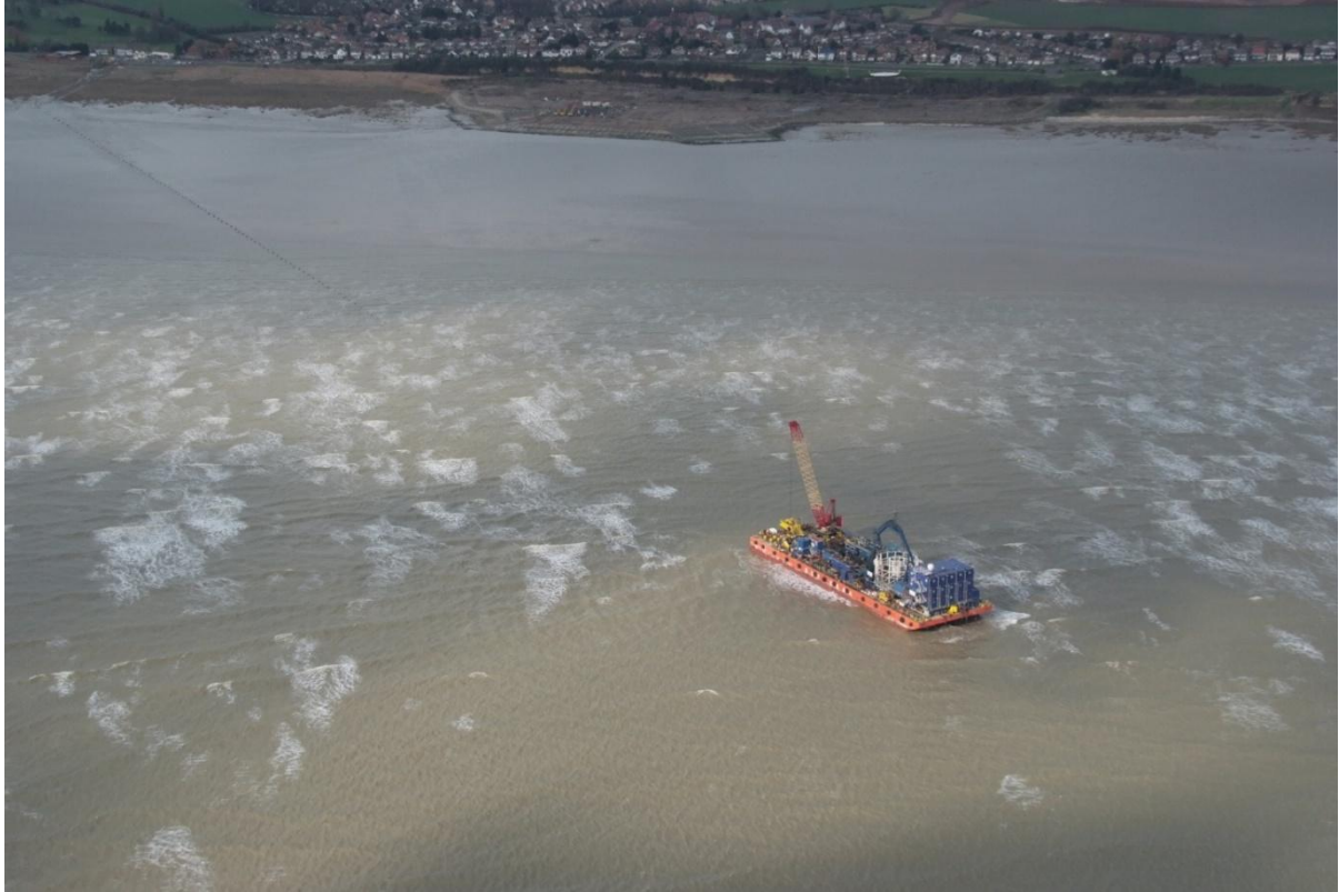
Figure 11. Cable Laying Barge in Pegwell Bay
