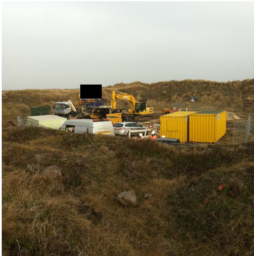
Figure 8. HDD Drilling “launch” site
