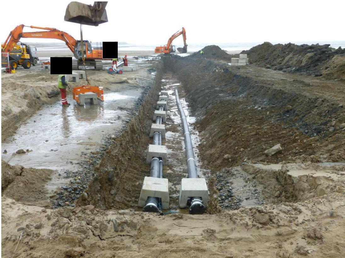
Figure 7. Pre installation of cable ducts.
