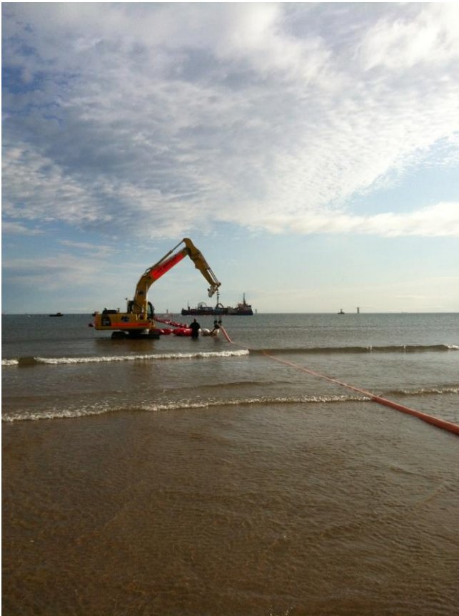
Figure 4. Removal of floats as cable is pulled ashore.
